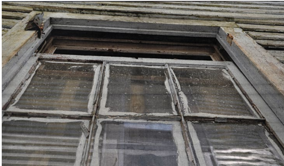
[23] (a) This deteriorated historic wood window was repaired and retained (b) in this rehabilitation project.
