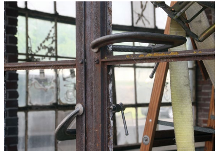
[20 a-d] The original steel windows in this industrial building were successfully repaired as part of the rehabilitation project (left).
